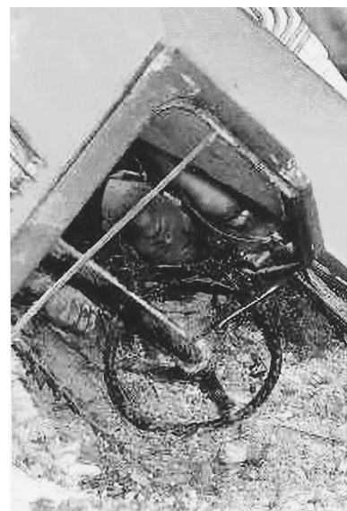
FIGURE 1. Case 1: The body was trapped upside down in the cabin of the excavator.
